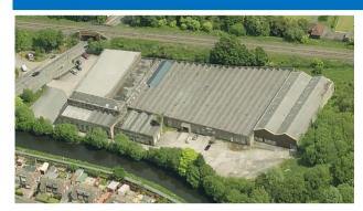
The works involved the demolition and site clearance of a 2-acre mill site; comprising a mixture of single storey 'North-Light' mill buildings; 2-storey offices and a more recent steel 2-span portal frame with asbestos cement cladding, plus additional amenity buildings, workshops and warehouse storage.
