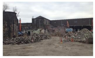
The structural demolition involved 4no hydraulic excavators equipped to demolition specification with fully protected cages and specialist attachments.
