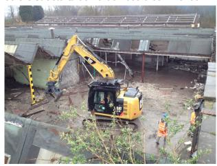
The aim was to completely demolish the buildings and structures on the site, including the removal of all the ground floor slabs and foundations, in order to leave a completely clear site ready for re-development.
