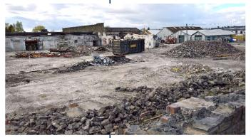
A large volume of materials were recycled on the site, including the reclamation of the roof slates; walling stone; mill floor stone flags; ferrous and non-ferrous metals, and timber from the roof structure.
