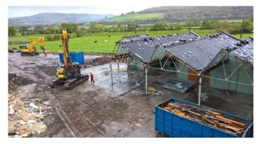
Crushing of all the hard rubble materials on site to produce c. 4000 tonnes of recycled aggregate for use by the Client in the permanent works.
