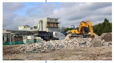
The works involved the demolition of a modern steel portal frame workshop structure and internal overhead gantry crane and including the breaking out and removal of the ground floor slab; concrete 'ring-beam' and pile-cap foundations.
