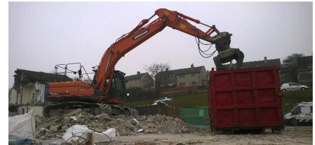
As the structural demolition took place all materials were loaded into HGVs and systematically removed from site for recycling.
