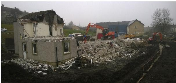
The aim was to completely demolish the buildings and structures on the site, including the removal of all the ground floor slabs and foundations, in order to leave a completely clear site ready for re-development of the new apartments.
