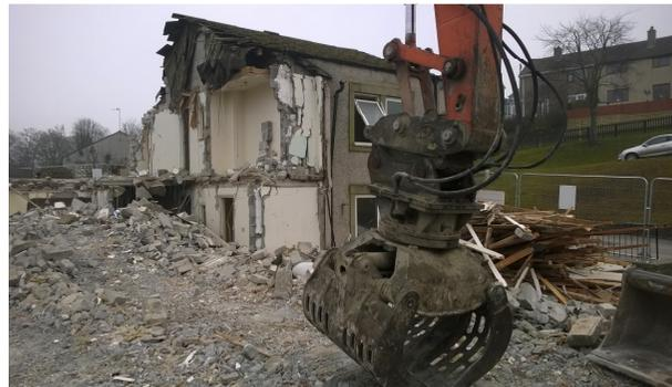
The soft-stripping process allows us to segregate all the waste materials and ensures that we maximise the amount of material that is recycled / reused. We currently aim to recycle c. 95-98% of all materials, and on this particular scheme even all the brickwork; blockwork; concrete slabs; precast floors; and structural foundations were all sent for crushing in order to produce recycled aggregates for use in other construction works.
